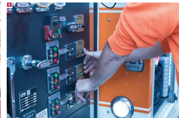
4 The final dump site arrangement comprised five dump tanks and delivered a 1,100-gpm flow. 5 Engine 54-4's operator primes multiple suction inlets at the same time.
